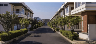
THE LAKE VIEW ADDRESS Mixed Residential Development | Phase I, Electronic City
